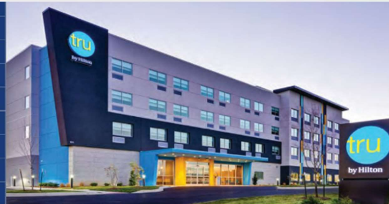
HAMCO IS DEVELOPING A TRU BY HILTON HOTEL NEAR THE BENNER PIKE I-99 INTERCHANGE.
